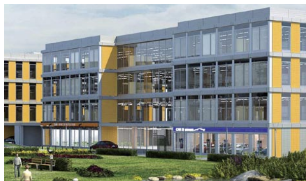
Enterprise Park, Kraków
